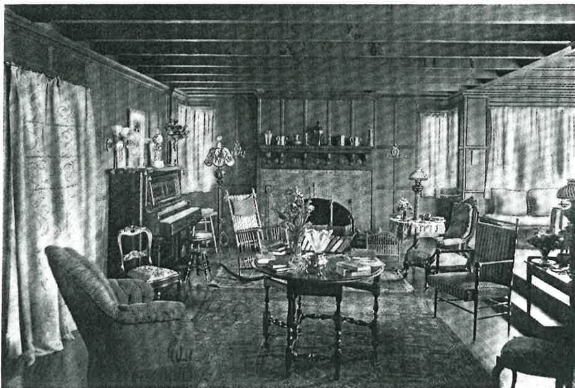
The Walls of the Living-room Are Paneled with Cypress, Stained a Soft Brown
