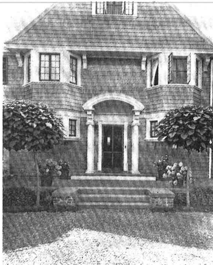
A Fine Doorway Gives a Distinct Character to the House
